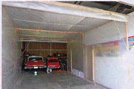
Our original plan was to bolt the booth together and take it down when not needed. As this area is normally used just for storage, we decided to add "roll up doors" at each end to make it a drive-through.
