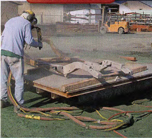
We started to clean the frame with a scraper and a wire brush, after a couple hours we came to our senses and hauled it to the local sandblaster.
