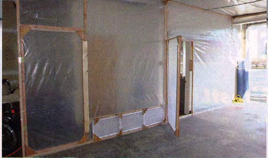
Two of the square frames were attached with spacers to each of our shop's sidewalls. We connected each set of side frames with more 2x2s and lengths of 1/2-inch conduit—the result is a 12x20-foot booth. We built a couple of doors in the sidewall of the booth from more 2x2s for access to the outside door and rest of the shop (note the filters in the wall).
