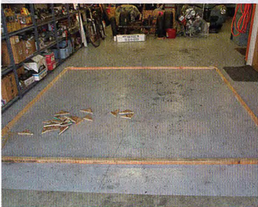
We've got so many parts and pieces to paint, so we decided to build a temporary paint booth. We used 2x2-inch lumber and built four frames that were 10-foot square.
