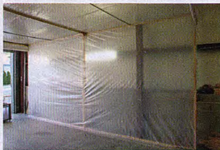
Here's one of the finished sidewalls. We mounted light fixtures outside the plastic to keep them clean. Along with the overhead fluorescents, the lighting in the booth is quite good.
