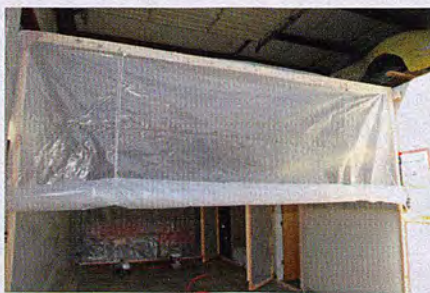
The ends were closed with plastic that was stapled to the top ends of the framework—then a 2x2 stapled to the plastic across the bottom. For access ropes and pulleys roll the plastic up like a window shade.
