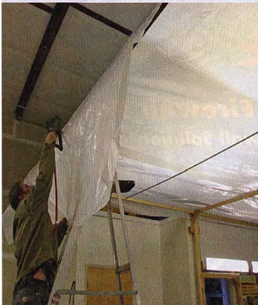
We picked up a 100-foot roll of 10-foot-wide 6-mil plastic to cover the roof of the booth as well as the sidewalls and stapled it in place.
